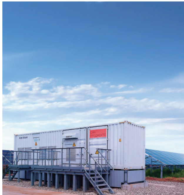
02 Utility Project in the Russian 300MW PV Plant
