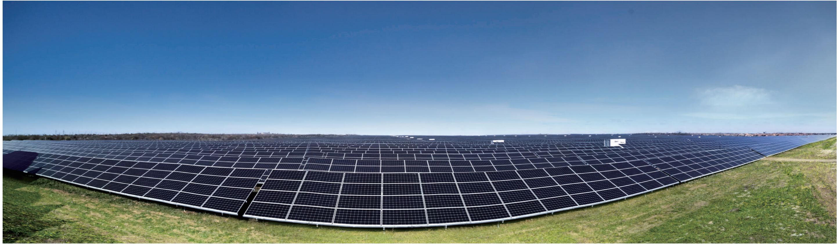
01 Utility Project in the Ukraine 240MW PV Plant
