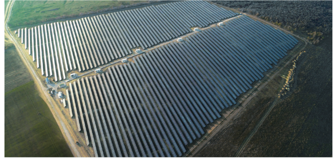
08 Utility Project in the Ukraine 15MW PV Plant
